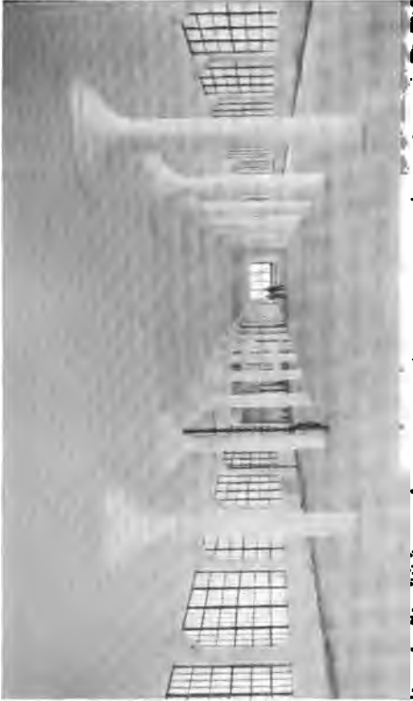
Fig. 2. Gray & Davis Plant, interior. The arrangement of this building is such as to give excellent illumination, the interior finish diffusing the light throughout the room. To the eye, the central bays appear practically as light as those at the sides.
